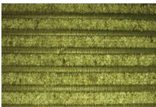
*Mould growing on heating coils*
