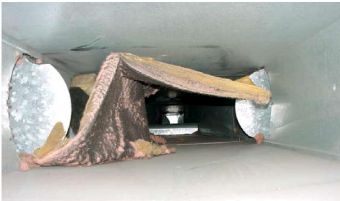
Section of insulation broken free in supply duct
