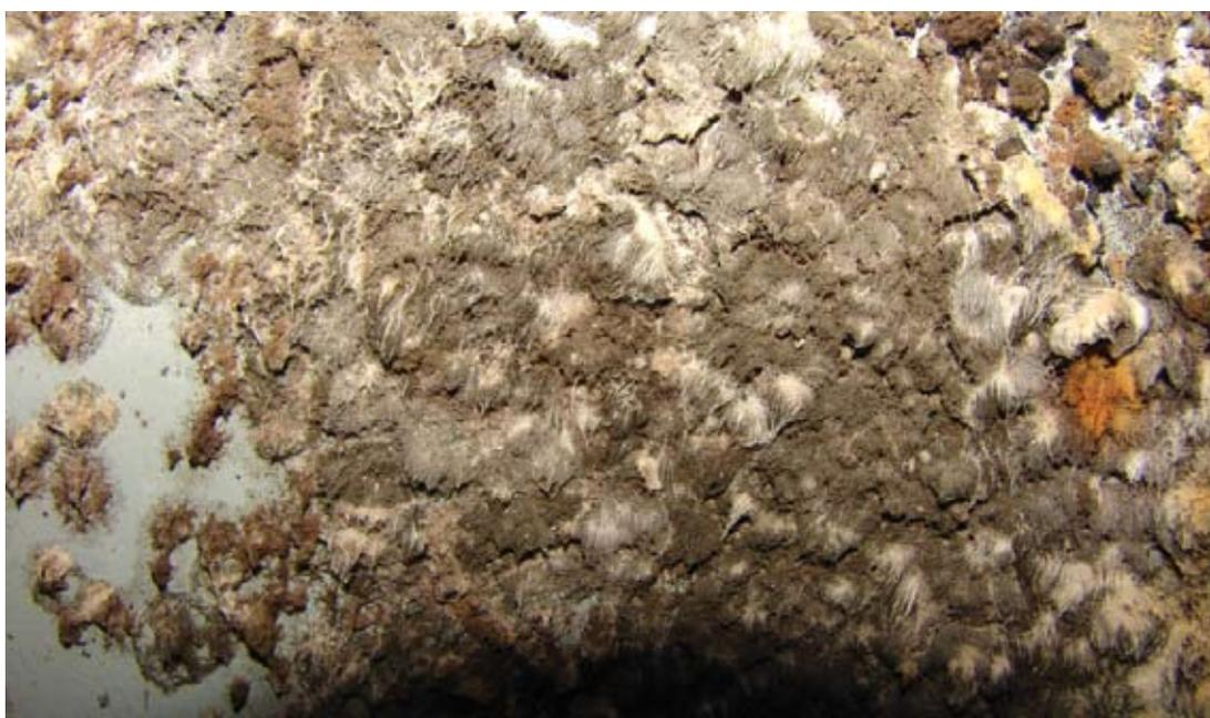
*Mould growing on a fan shroud*
