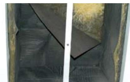
Exposed fibreglass insulation in cushion head
