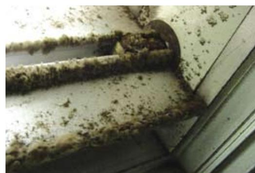
*Mould growing on a volume control damper*
