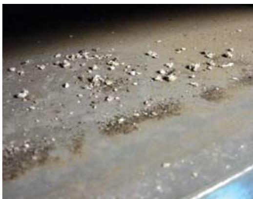
*Particles of sprayed asbestos insulation that has travelled down a supply air duct*
