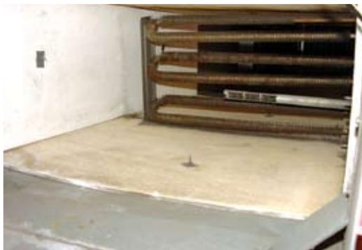
*Insulation surrounding inline electric heating elements in buildings built pre 1980 generally contain asbestos.*
