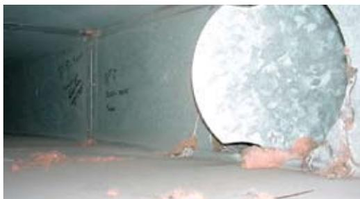
Fibreglass particles in supply duct from air handling unit insulation
