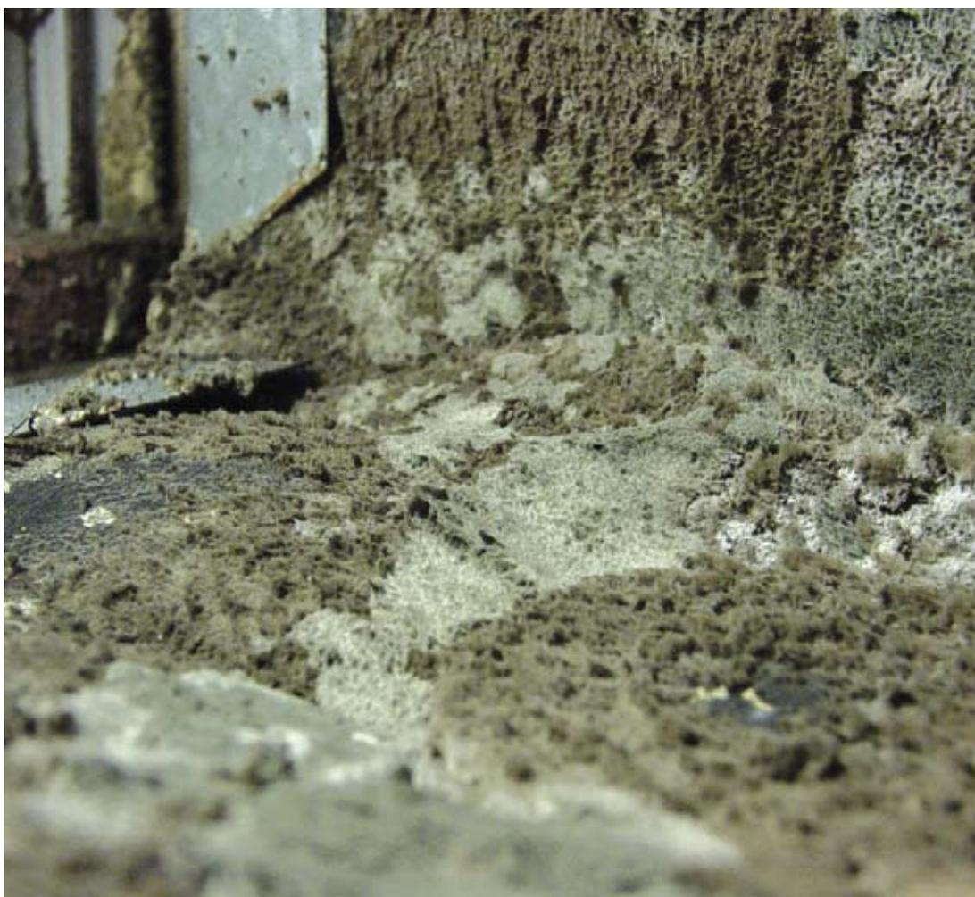
*Mould growth on internal insulation*
