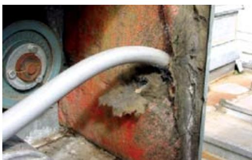
Deteriorated insulation within fan coil unit
